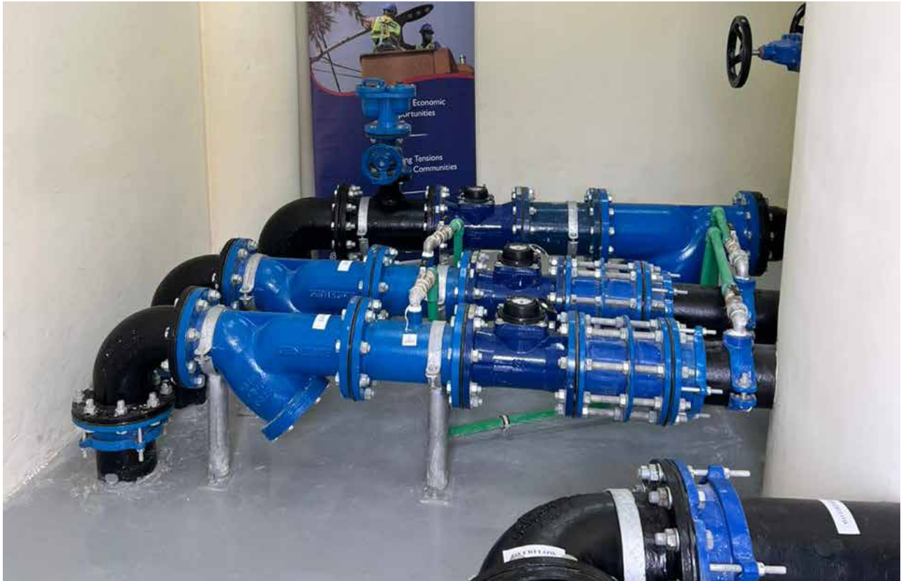
The installation of the wastewater tank pipes in Bqosta
