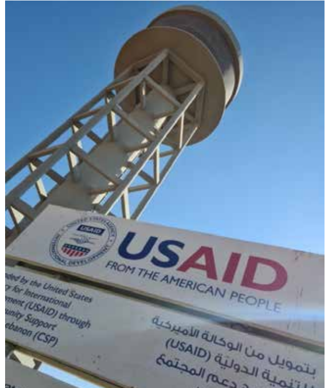
Construction of the 300m 2 elevated water tank in Talia
