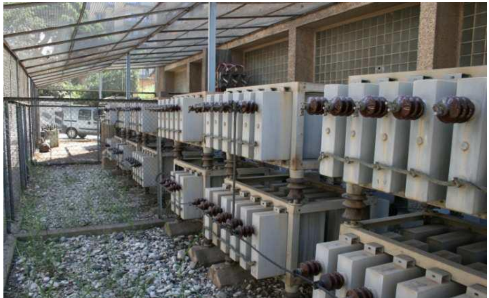
Capacitors & transformers piles: Bauchrieh
